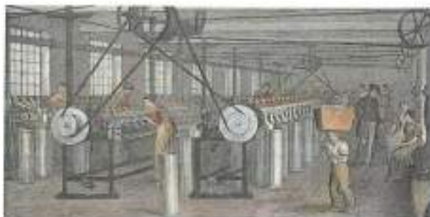
Figure 34: Inside a cotton mill at the peak of the development of Cottonopolis.
